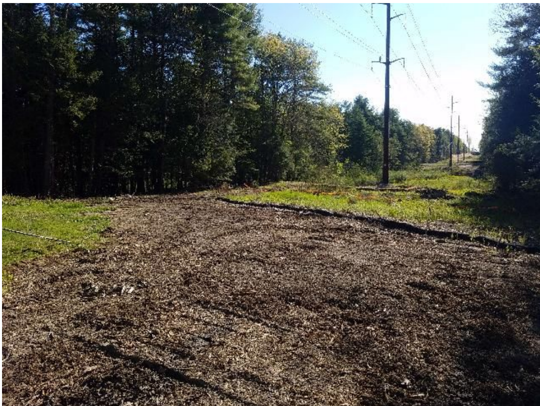
Fig 2: Removing timber mat access road to Str. 68. Viewing east. (05-21-20).
