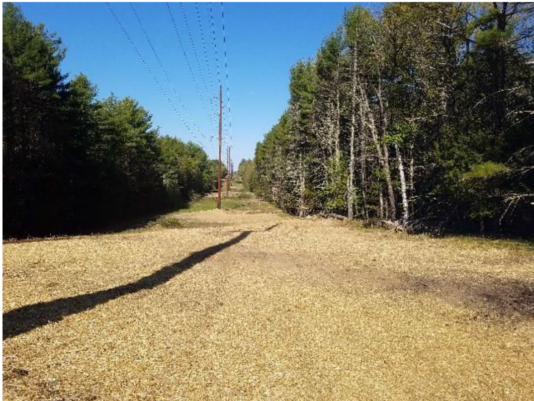
Fig 4: Strs. 72 & 71 work areas restored. Viewing west. (05-21-20).
