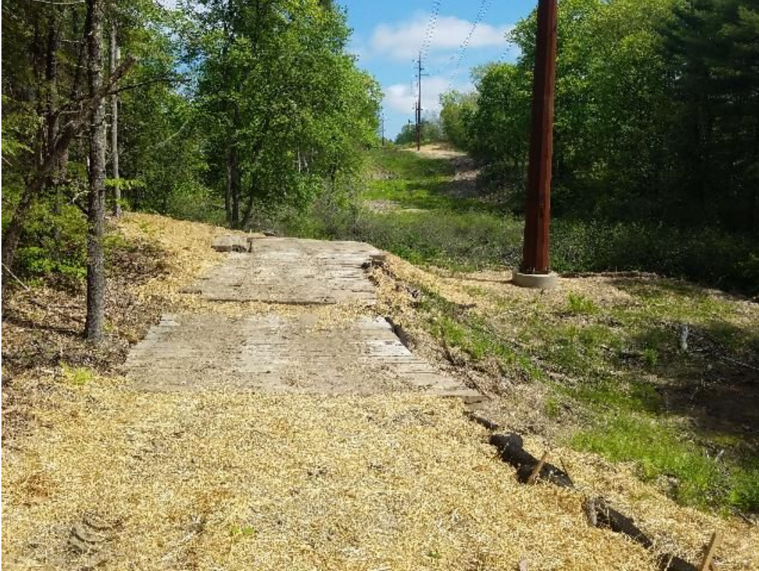
Fig 11: Temporary road installed to access Str. 28. Viewing north. (05-26-20).
