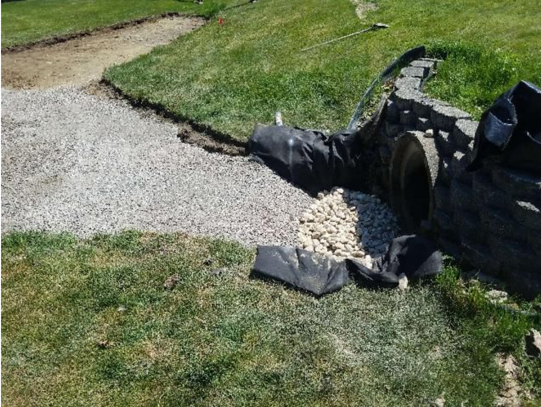
Fig 9: Repairing seepage area on the Veitas property. Viewing northeast. (05-56-20).
