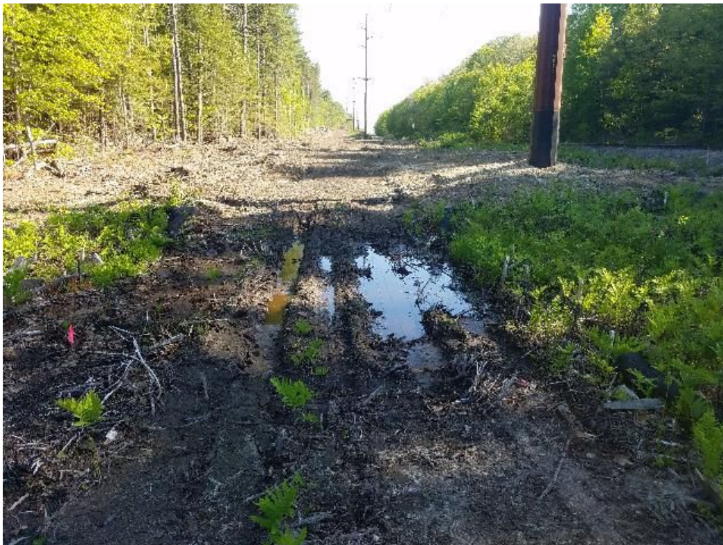
Fig 14: Rutting in wetland DW79, near Str. 15. Repairs will be made during restoration. Project wide restoration is underway. Viewing north. (05-27-20).
