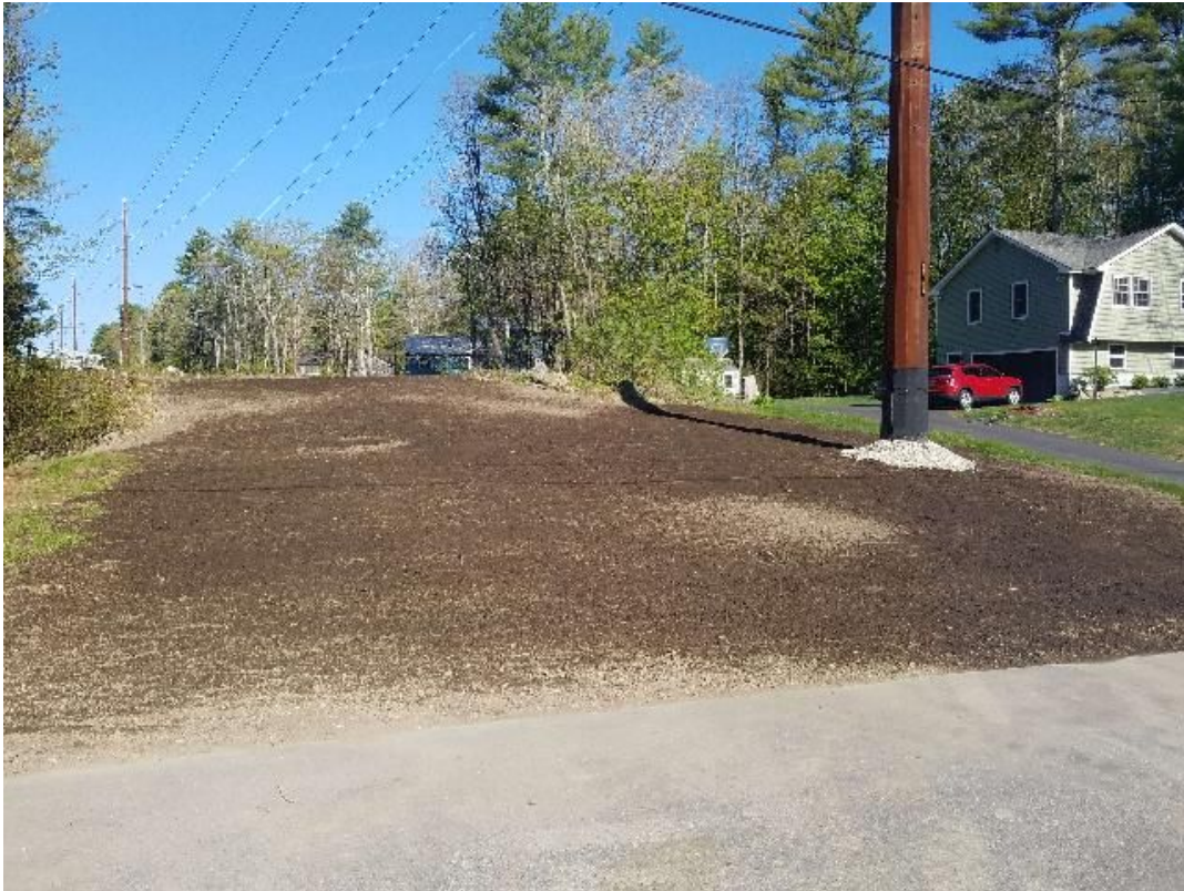
Fig 1: Str.67 final restoration. Viewing west. (05-21-20).
