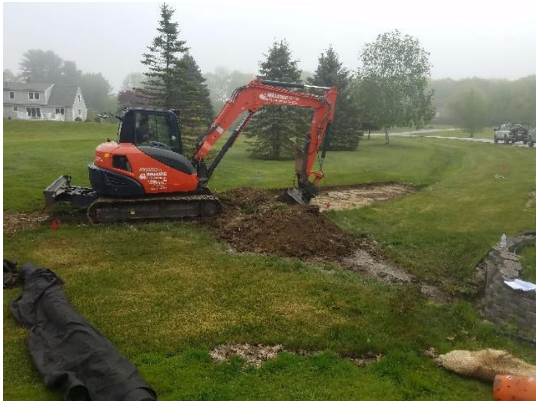
Fig 8: McCourt repairing seepage area on the Veitas property. Viewing northeast. (05-56-20).
